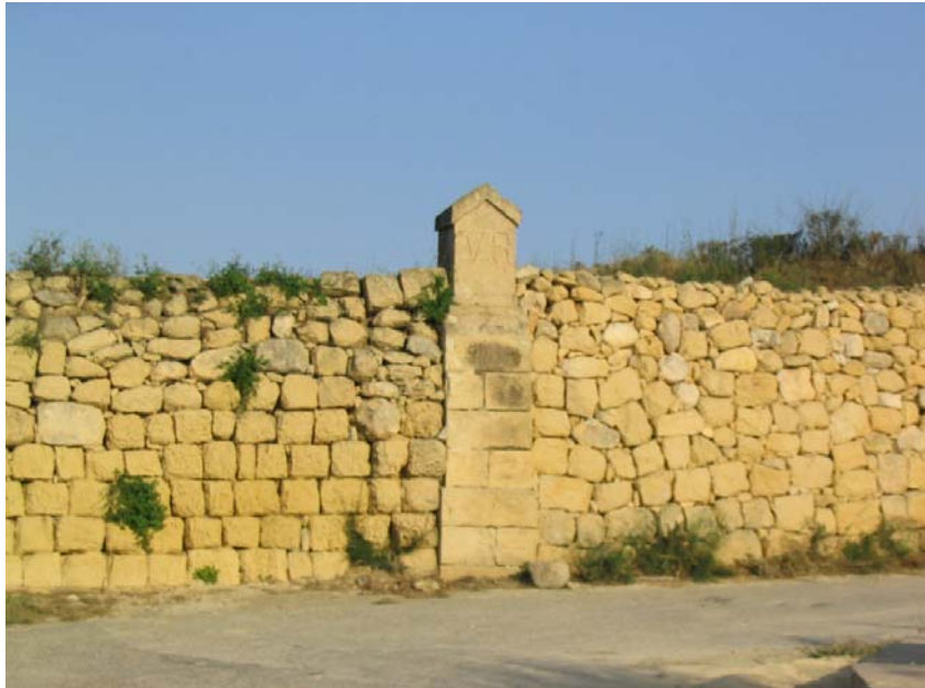
Photo 5: Impressive, well weathered, Victorian property marker
